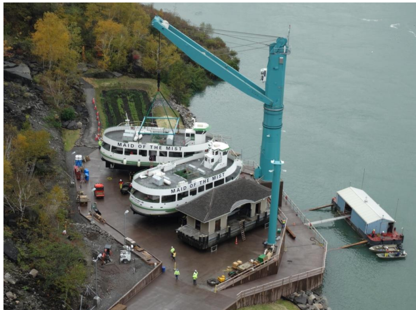
New Drydock after lifting the boats out of the water
