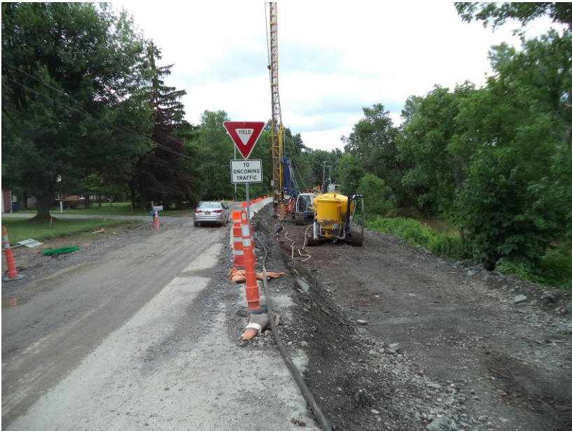
View of Dry Soil Mixing Operations
