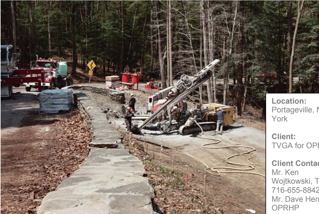
Drilling Anchors into Slope Face
