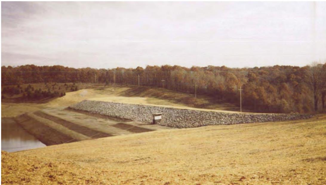
**Figure 6. Upstream slope after completion of remedial construction**
